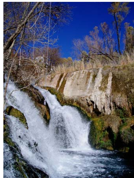
Fossil Creek Dam after restoration
